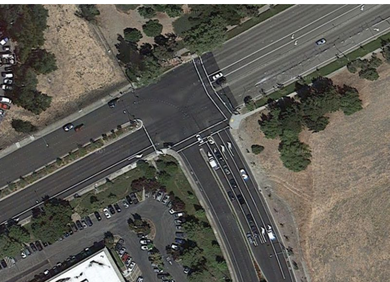
Figure 3. Mitigating auto LOS to D has created vast amounts of asphalt that are unused for most of the day, as shown by this eight-lane arterial.
