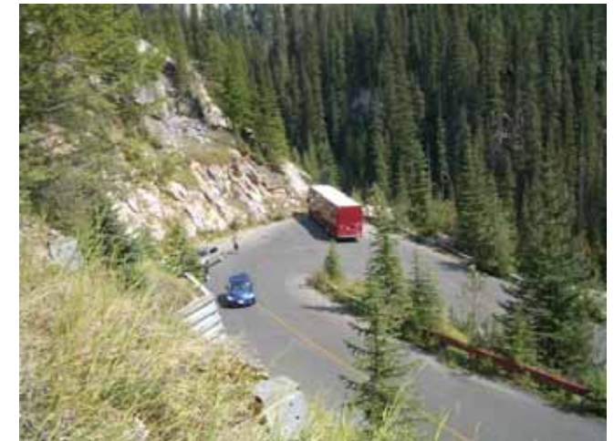
1. Bus using the holding bay provided at each switch back to commence its reverse ascent
