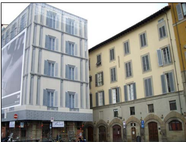
Spot the Scaffolding
